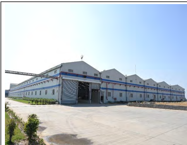
MANUFACTURING PREMISE ENTRY
